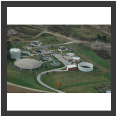
Wastewater Treatment Plant
