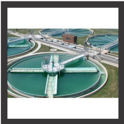
Effluent Treatment Plant
