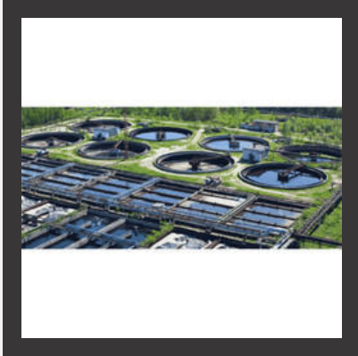
Water Treatment Plants
